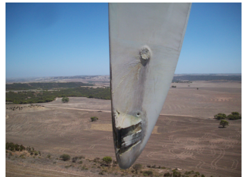
Figure 2: Damage to a wind turbine tip due to a lightning strike.
