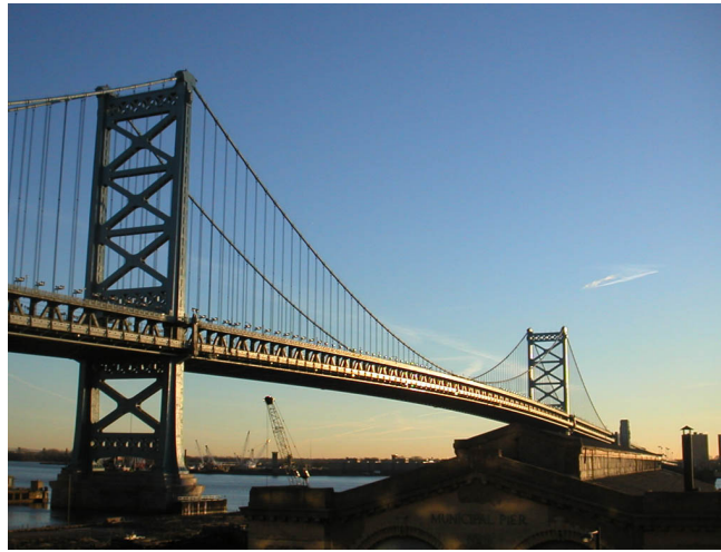
Figure 10. Instrumented Ben Franklin Bridge spans the Delaware River
