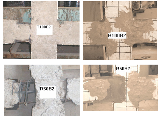
Figure 3. Specimens before and after rehabilitation
