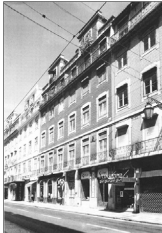
Figure 1 – Analyzed building (Prata Street, 210 to 220, in Santos[4])
